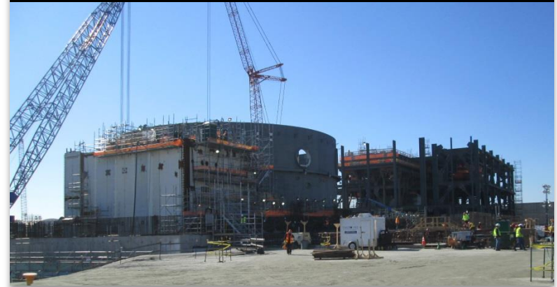
V.C. Summer Unit 2 NI and Turbine Building, March 2016
