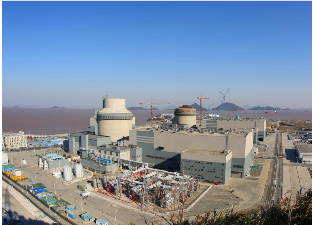
Photo © Sanmen Nuclear Power Company Ltd/ All rights reserved.
